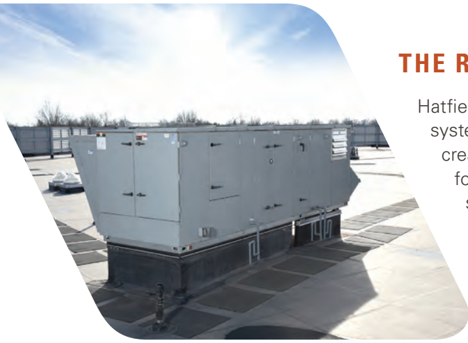
A Valent VPRC unit installed on the rooftop at Hatfield Elementary
